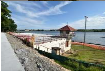
Figure 39. The photograph was taken on the southern pathway of Memorial Park looking south – east towards the boatshed. What is evident is the replace roof with metal deck which is unsympathetic to the c.1930 structure and should be removed. Source: Celeste Greeves, December 7 th 2022.
