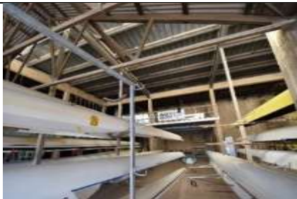
Figure 47. The photograph was taken at the south – east entry of Grafton Rowing Club Boatshed looking north – east. Evident in the image is the concrete structure to the c.1930 building which is to be retained in the development. It should be noted that it is evident that the roof covering (concrete deck) has been replaced with metal deck roofs. Source: Celeste Greeves, December 7 th 2022.
