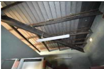
Figure 56. The photograph was taken in Grafton Rowing Club Boatshed amenities. Evident is the modified roof structure with infill roofing to cover the amenities. Source: Celeste Greeves, December 7 th 2022..
