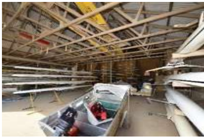
Figure 46. The photograph was taken at the south – east entry of Grafton Rowing Club Boatshed looking north – west. Evident in the photograph is the timber truss rafters that have utilised providing a roof structure to the shed extension. Source: Celeste Greeves, December 7 th 2022.
