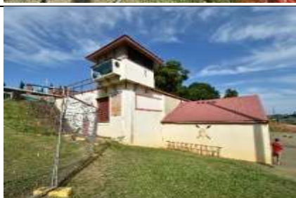
Figure 30. The photograph was closer up to the Grafton Rowers boatshed illustration, the two external phases of construction, c.1930 and c.1996. Evident is the previous openings now enclosed to the c.1930 shed. Source: Celeste Greeves, December 7 th 2022.
