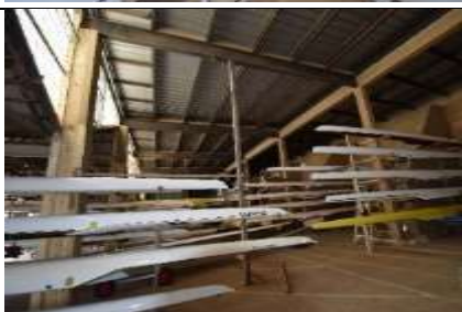
Figure 48. The photograph was taken at the south – east entry of Grafton Rowing Club Boatshed looking north – west. Evident in the photograph are the changes to the roof structure with timber rafters to support the steel decking to the roof, and additional steel column (centre of the picture). Source: Celeste Greeves, December 7 th 2022.
