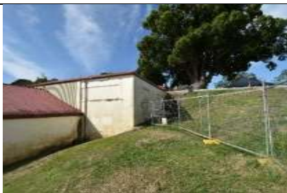
Figure 42. The photograph was taken looking at the south and eastern façade to the c.1930 boatshed building and the c.1996 extension added to the original structure. What is evident in the image is the infill to the window opening to the c.1930 building structure. Source: Celeste Greeves, December 7 th 2022.
